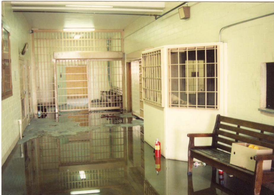
The control center area of SCI Camp Hill.
